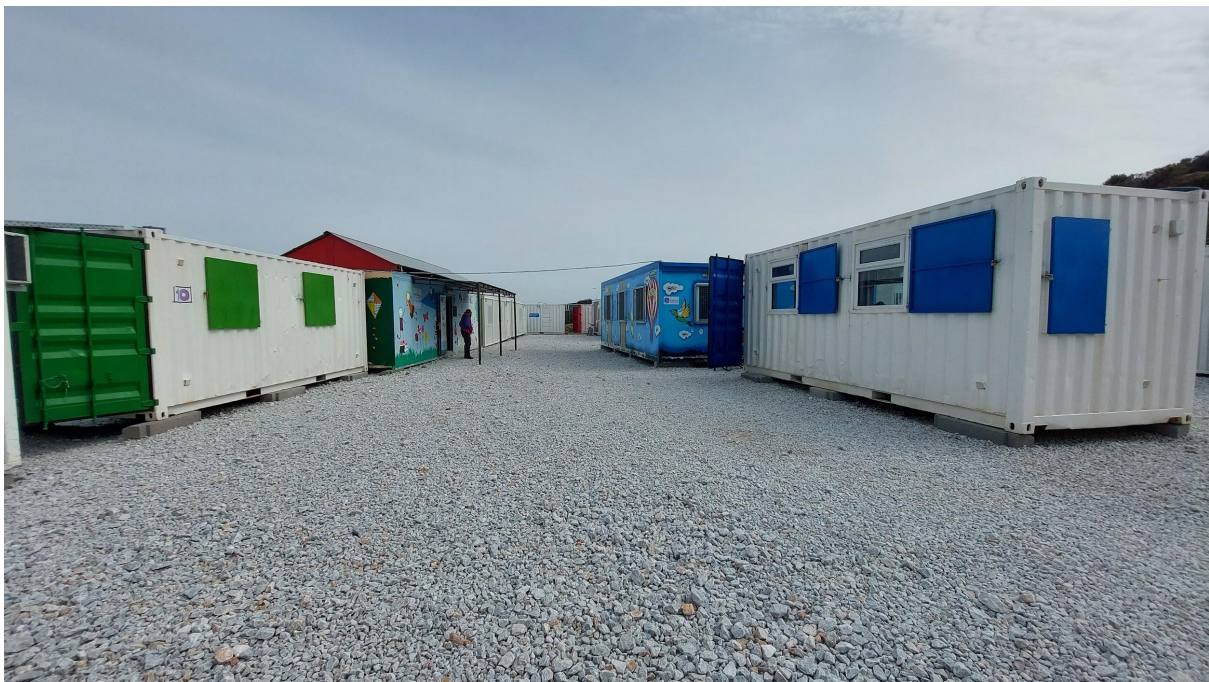
Education center inside Mavrovouni camp before our construction works
